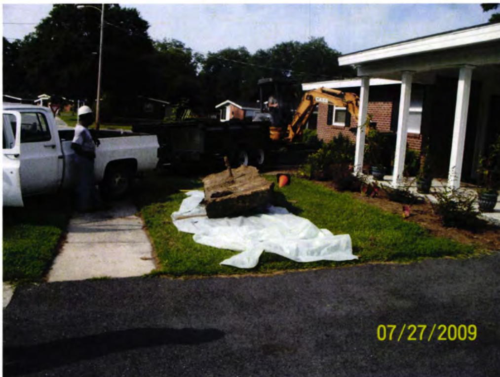
Picture 2: Concrete lid removed from top of UST 1393 Dove-2
